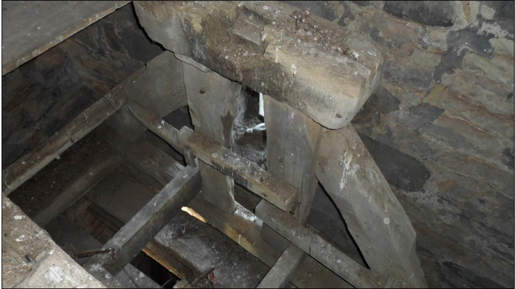
Figure 3: Truss D, photograph taken from the north-west
