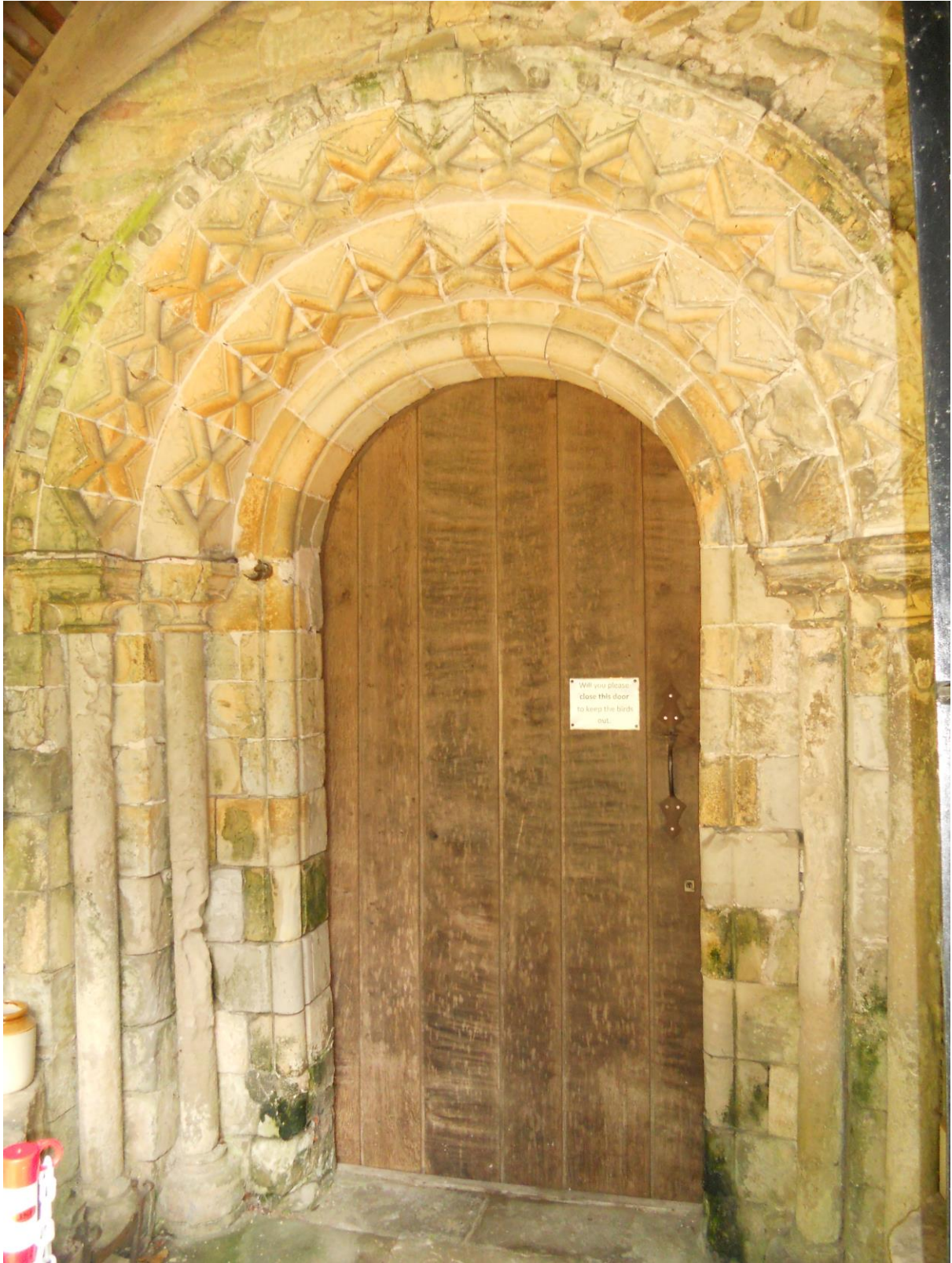
Figure 6: External view of south door with replacement door shut (DM)
