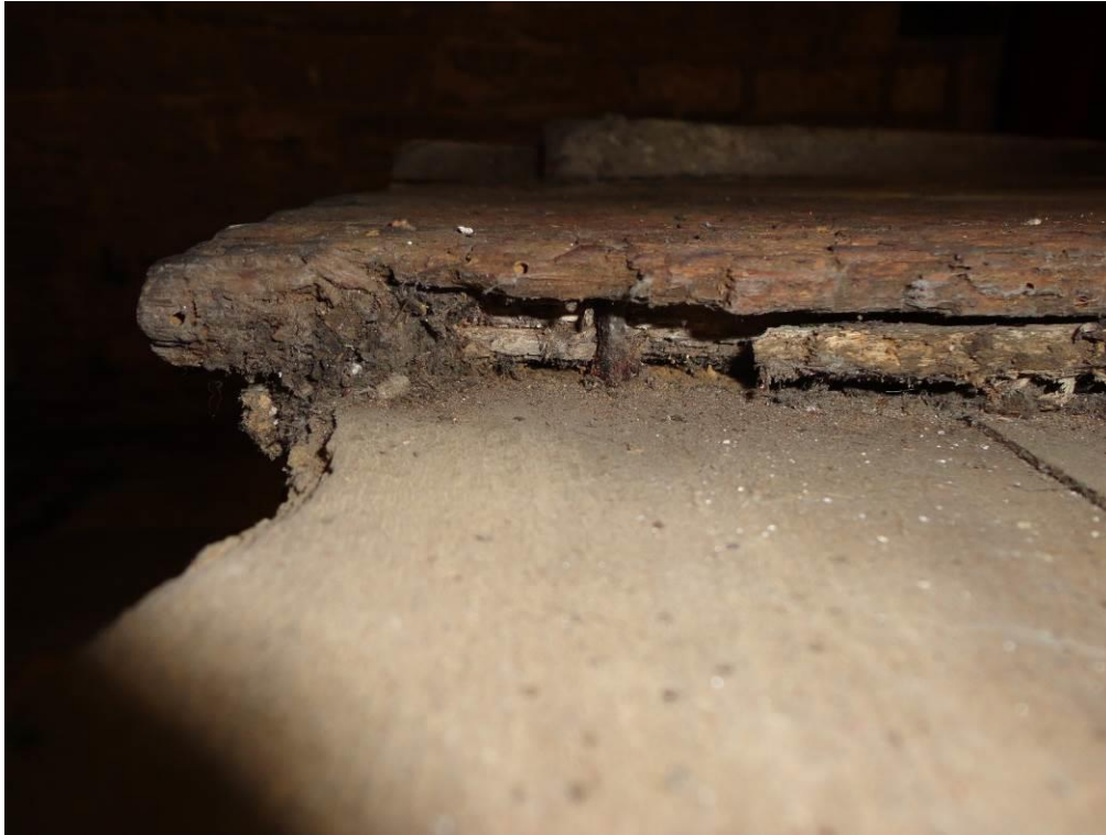
Figure 4: Edge of the bottom of board 3 showing the stopped loose tongue groove at bottom of board from the hinge side (DM)
