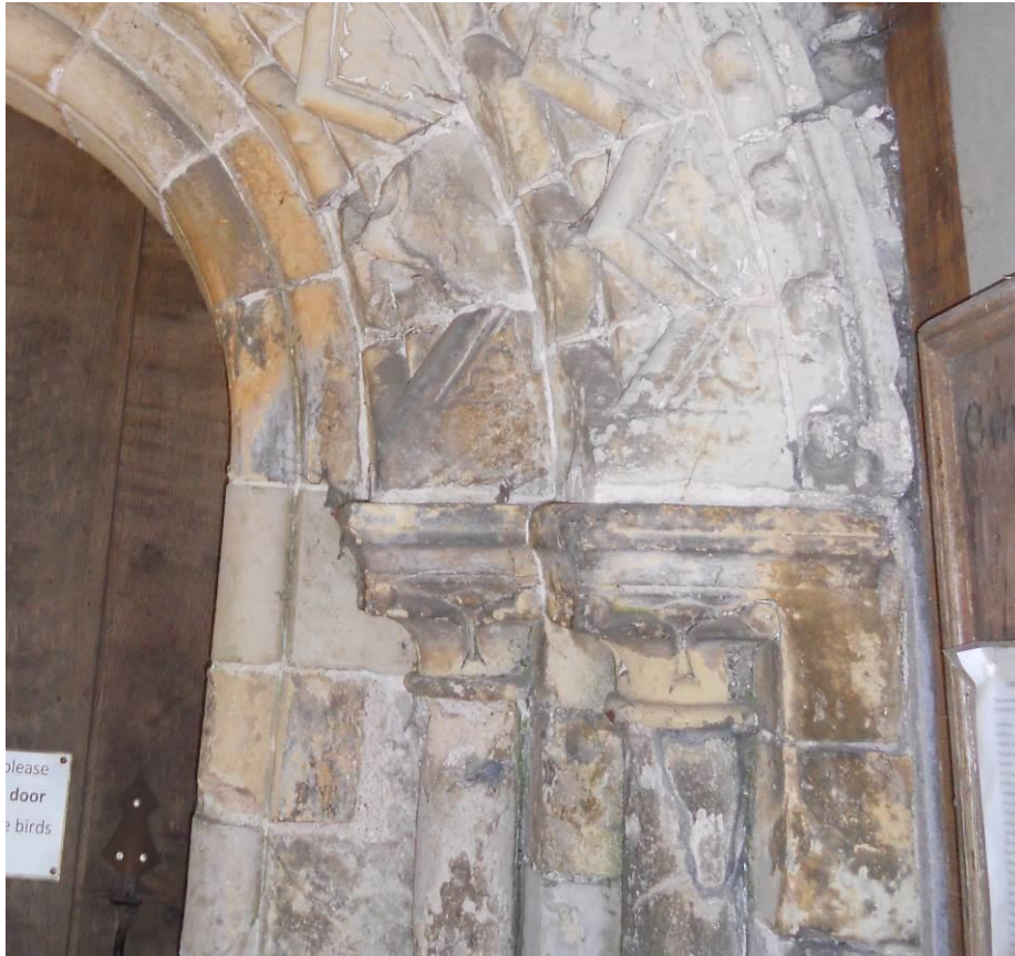
Figure 7: Detail of stonework shafts and capitals with arch (DM)
