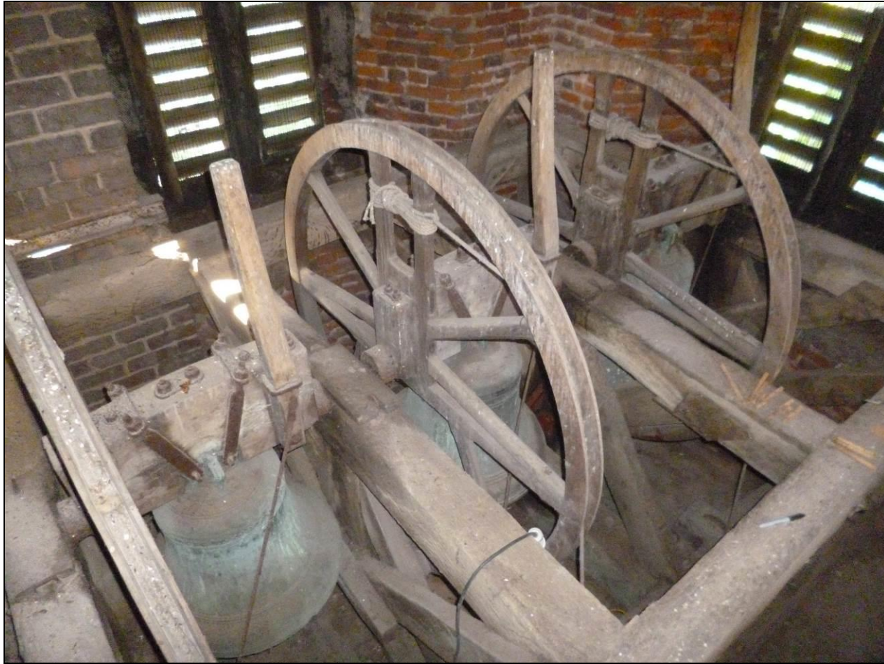
Figure 3: The bellframe, photograph taken from above
