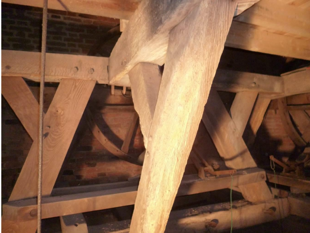
Figure 3: The bellframe, photograph taken from the west
