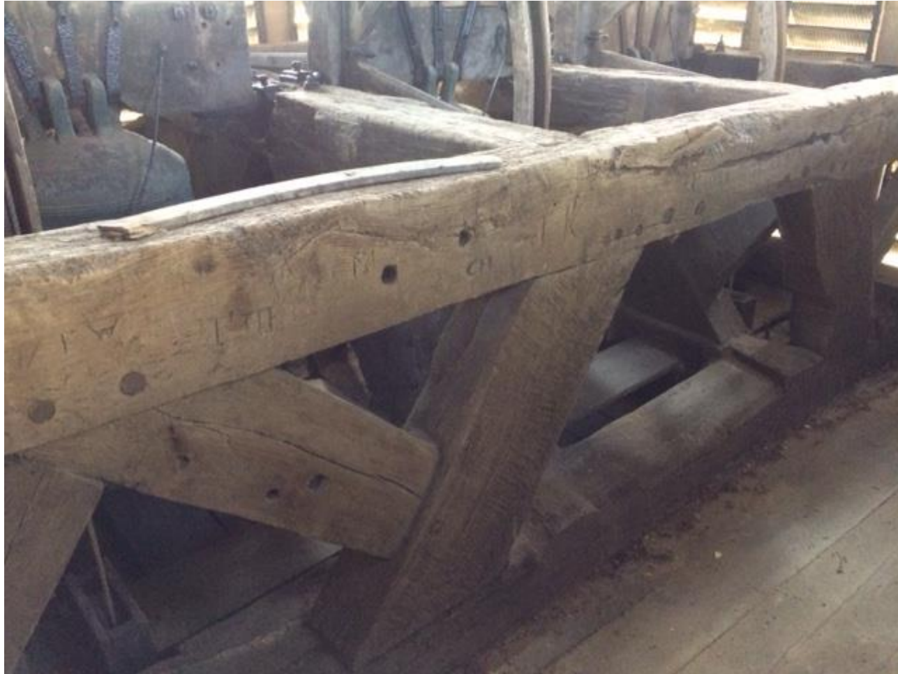
Figure 4: The bellframe, photograph taken from the north-west
