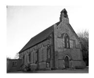
buttressed. At the east end is the apse which houses the Sanctuary. At the west end there is a large gallery. On the south side of the apse is a small vestry. The tiled roof of the nave is high pitched, and is supported by double hammer beams. Originally there was a stone cross surmounting the eastern apex of the roof, whilst at the west end the small belfry remains.
