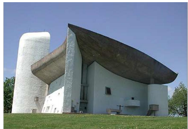
An example of international style: The chapel of Notre Dame du Haut in Ronchamp, France, designed by Le Corbusier 1954/5.
