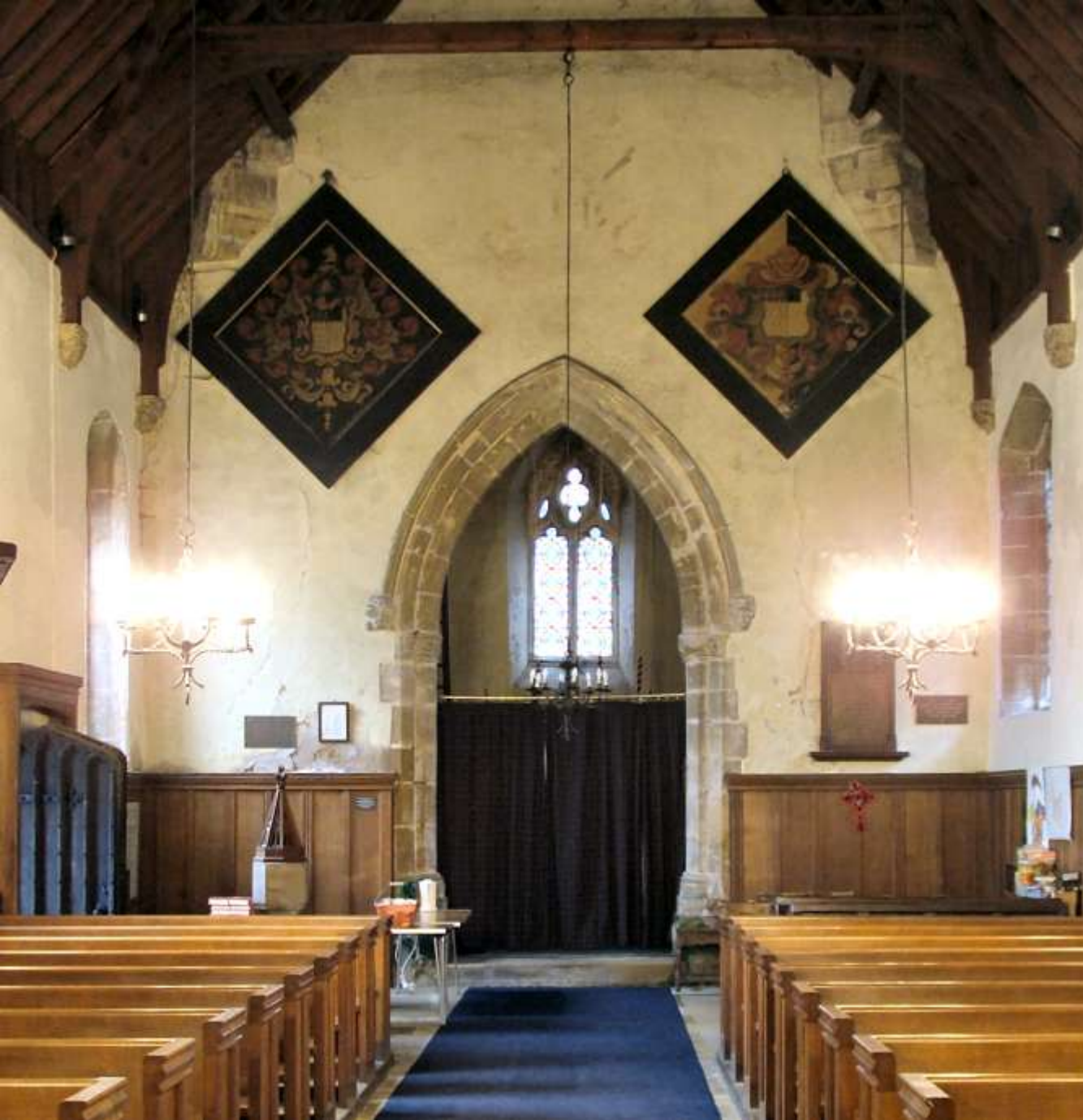
Averham: view west over tower arch
