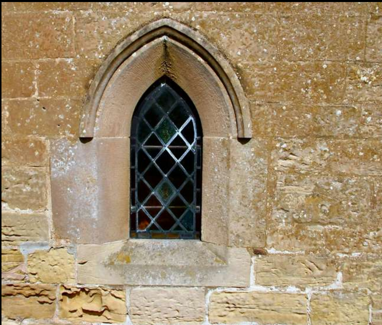
C19th window set into earlier medieval stonework
