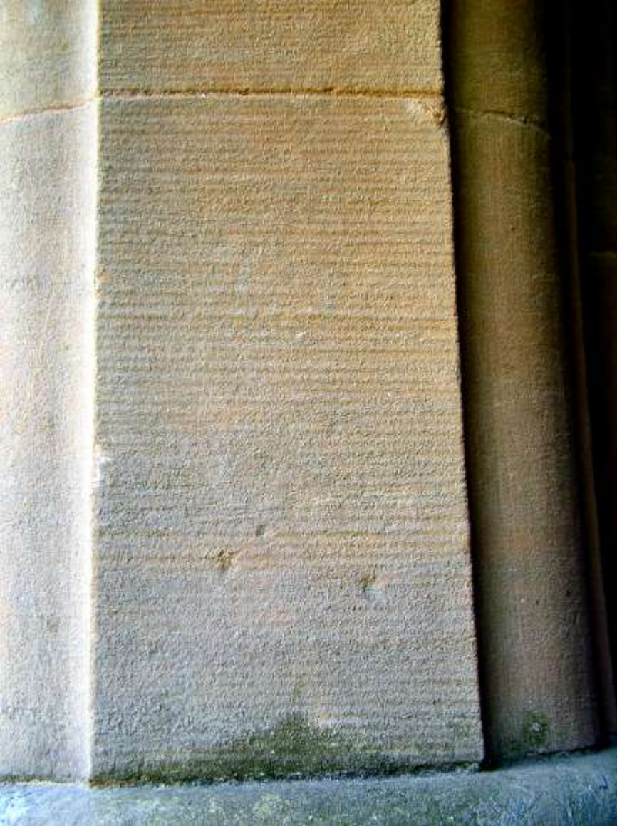
Typical late C19th tooling – note the regularity and length of tooling
