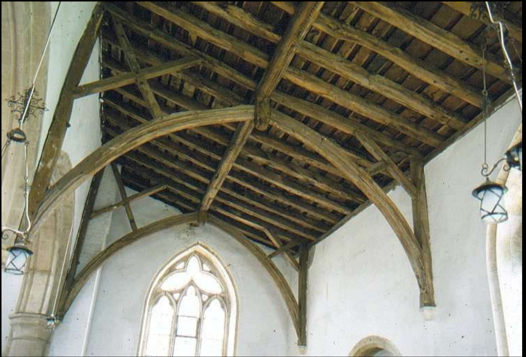
Orston, Notts. C14th N. aisle roof
