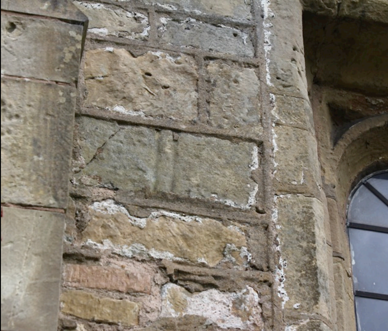
Norton Cuckney – north wall of chancel, fragment of shaft
