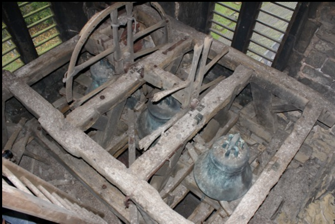
North Leverton: 3-bay Elphick 'W' frame, post- medieval
