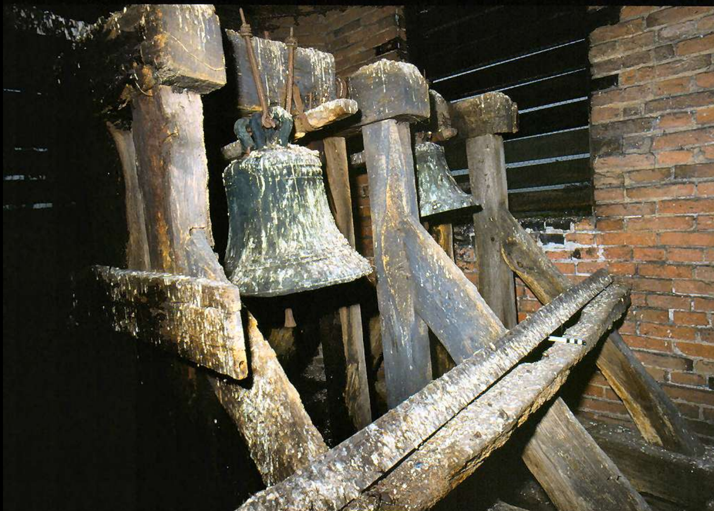
Morton: Pickford type 3.E variant short-headed bellframe formerly in C18th tower. Undated but probably from previous church.
