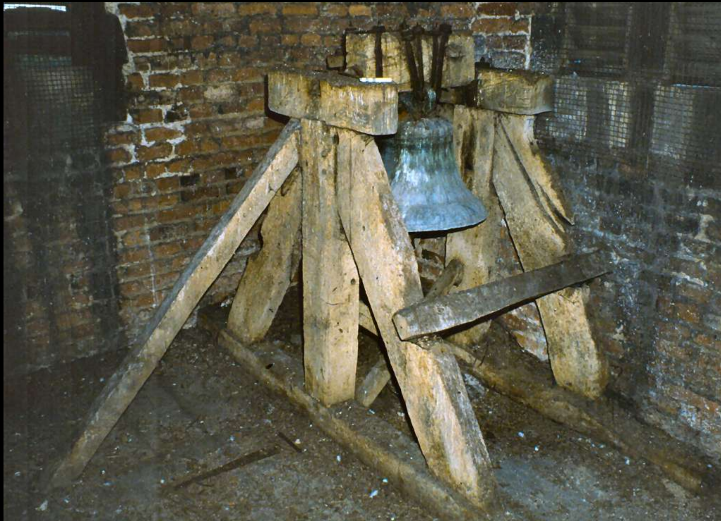
Carlton-on-Trent: short-headed frame (Elphick 'K' / Pickford 3.D. variant) in a C19th tower
