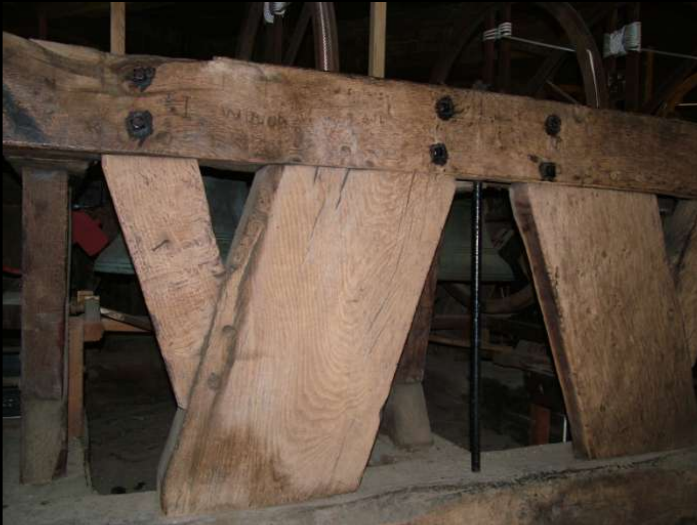
Southwell Minster: bell frame of c. 1720 Elphick type 'V'; Pickford type 6.B
